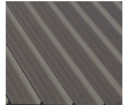
ROOF AEP SPAN - STANDING SEAM METAL ROOF
